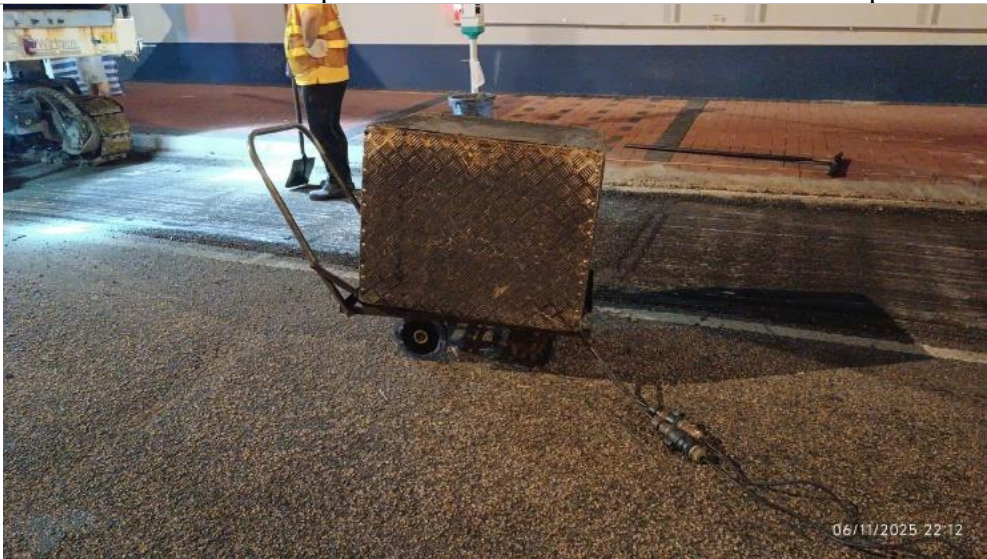
Acoustic enclosure was provided for portable generator’s operation.
