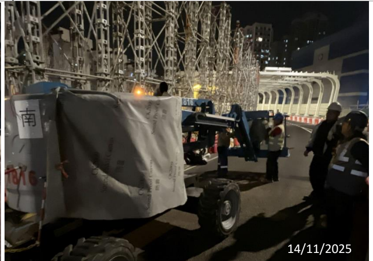
The power generating parts of the PMEs were covered with acoustics sheds.
