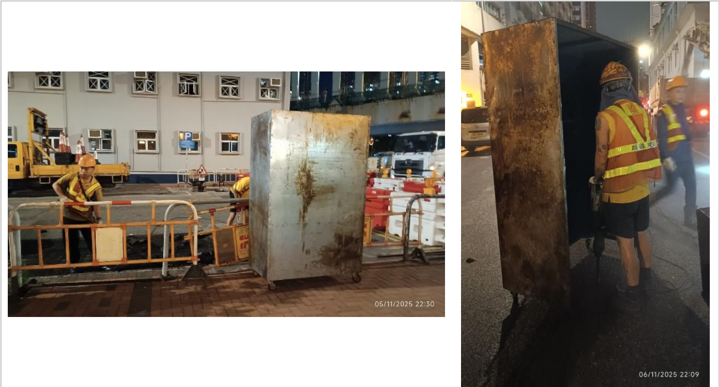
Acoustic enclosure was provided for electric hand-held breaker’s operation.
